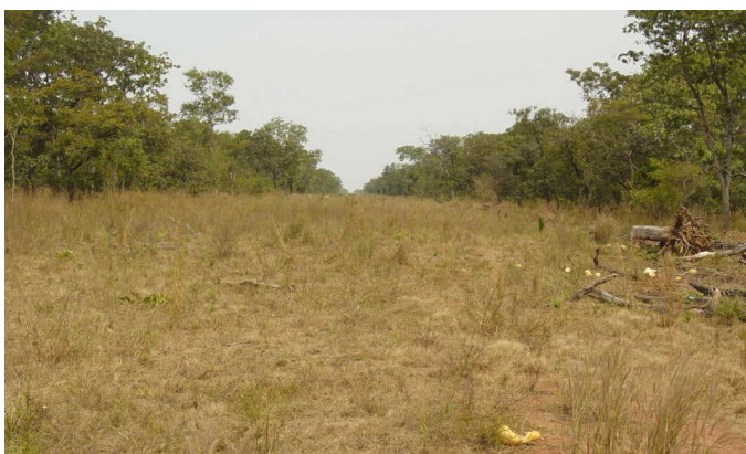
Figure 6D. A view of the reclaimed pipeline easement in the wooded savanna zone in southern Chad after the first rainy season.
