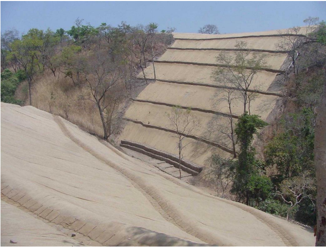
Figure 5B. Extensive use of vegetative matting and diversion ditches was required to control erosion in high relief areas in northern Cameroon.
