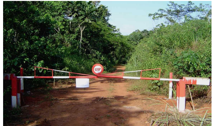
Figure 4E. A locked gate placed on a pre-existing road retained for pipeline maintenance and emergency response purposes in an induced access management area.
