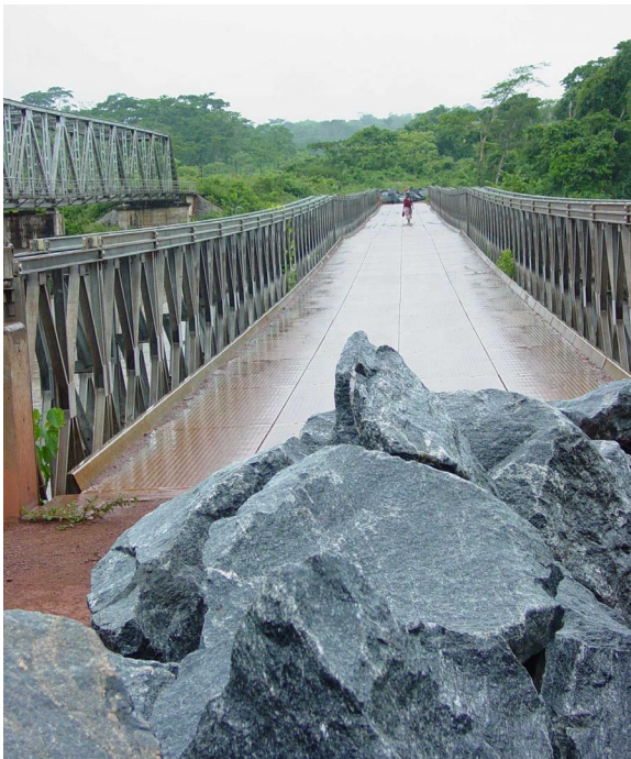
Figure 4C. A boulder pile placed at the end of a temporary bridge over a river in an induced access management area to prevent vehicular use of the bridge until it was removed.
