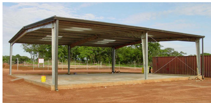
Figure 9A. One of the Project's waste storage buildings.
